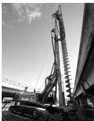
Vibro-Pile works at Australia's Monash Freeway upgrade project.
