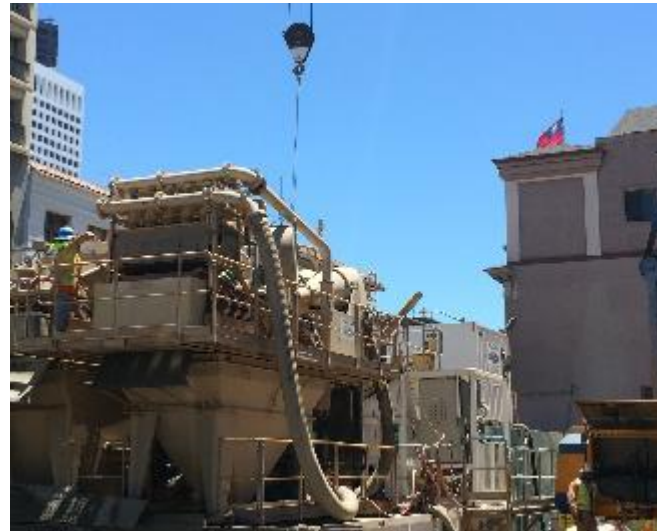
San Francisco Light rail
