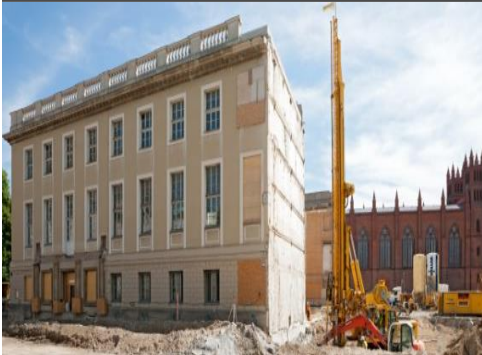
Complete excavation pit Berlin State Opera House, Germany
