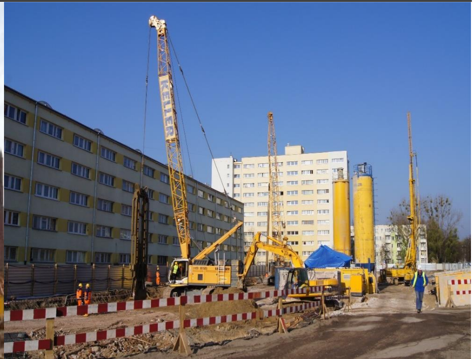
Diaphragm walls Nowy Swiat Financial Centre, Warsaw, Poland
