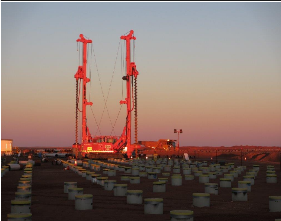
Piling, on-shore LNG processing plant Wheatstone, Western Australia
