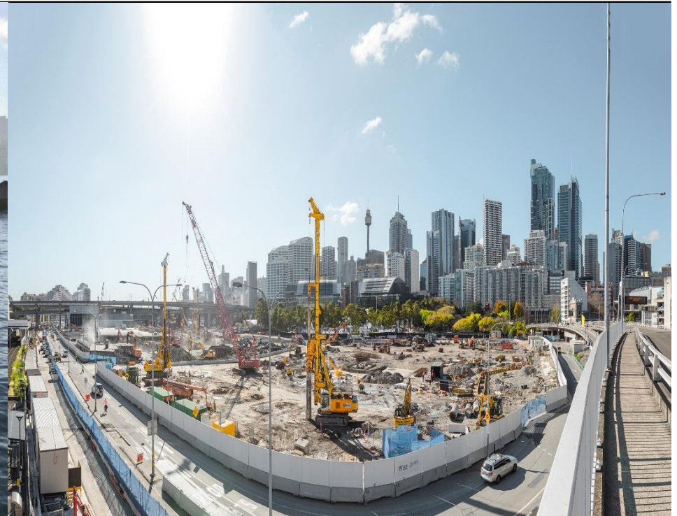
Various categories of piling Darling Harbour Live, Sydney
