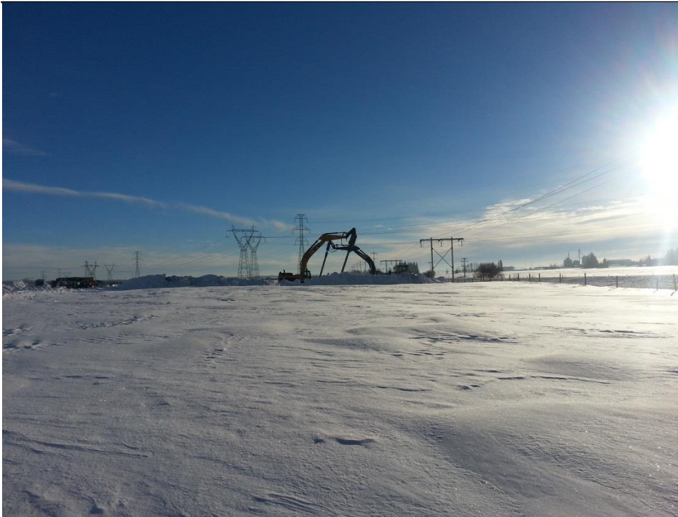
Piling, transmission lines
