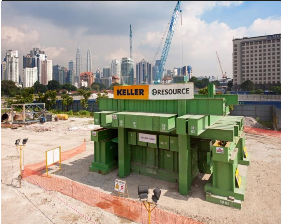
Load testing, mixed-use development Kuala Lumpur, Malaysia
