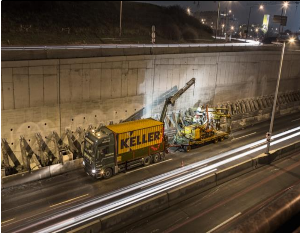
Soil anchors, highway repairs A23 Bypass, Vienna
