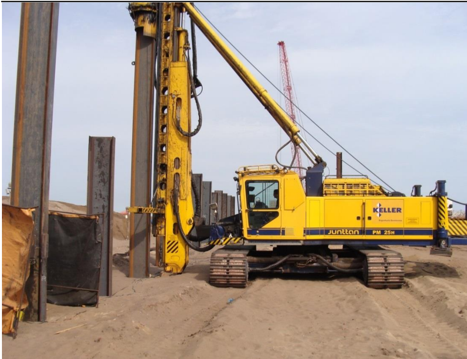
Piling, port development Rio de Janeiro, Brazil
