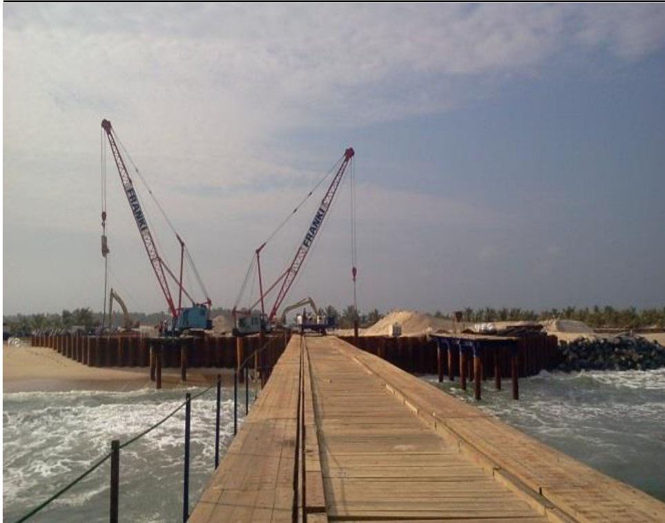
Piling, coastline remediation
