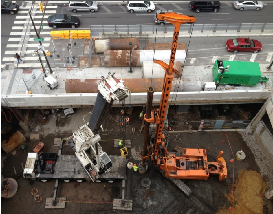
Piling, residential tower
