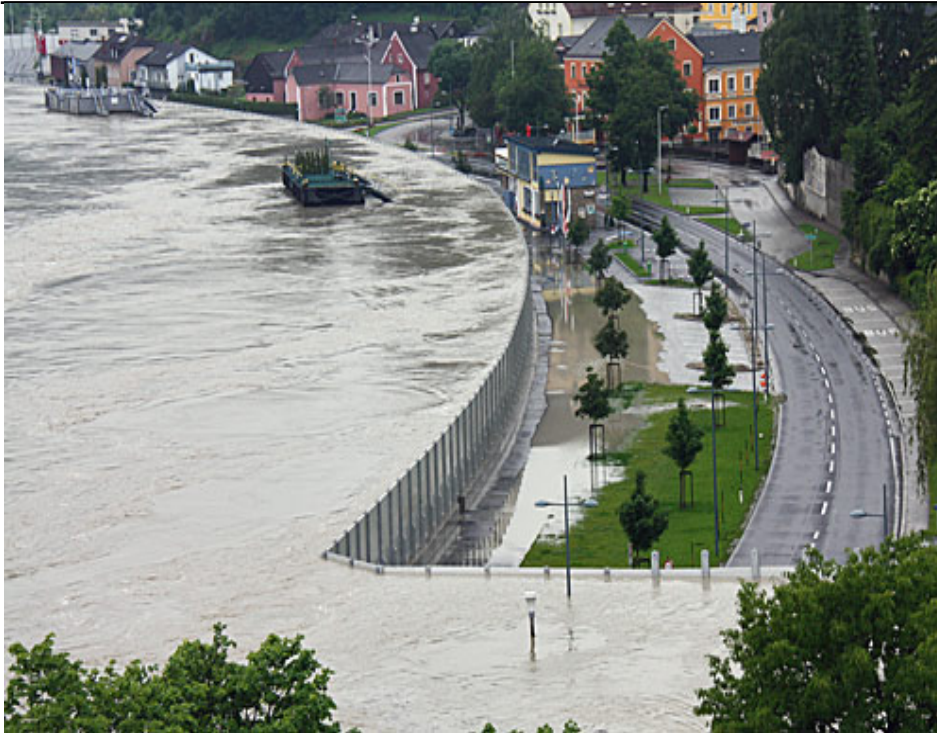
Piling, river flood protection
