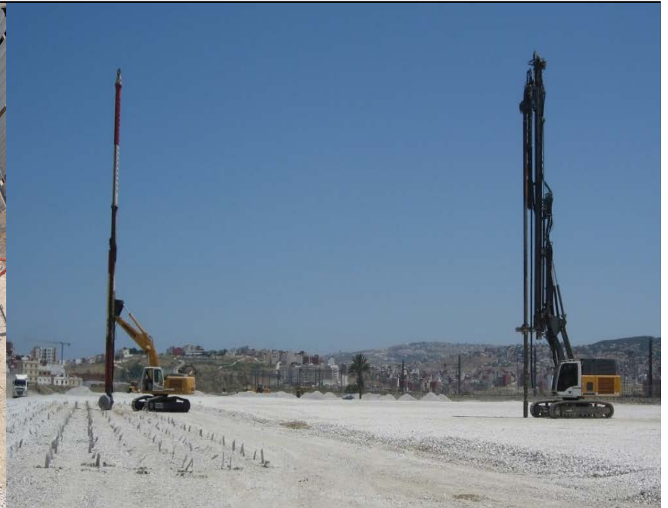
Ground improvement, rail maintenance workshop
