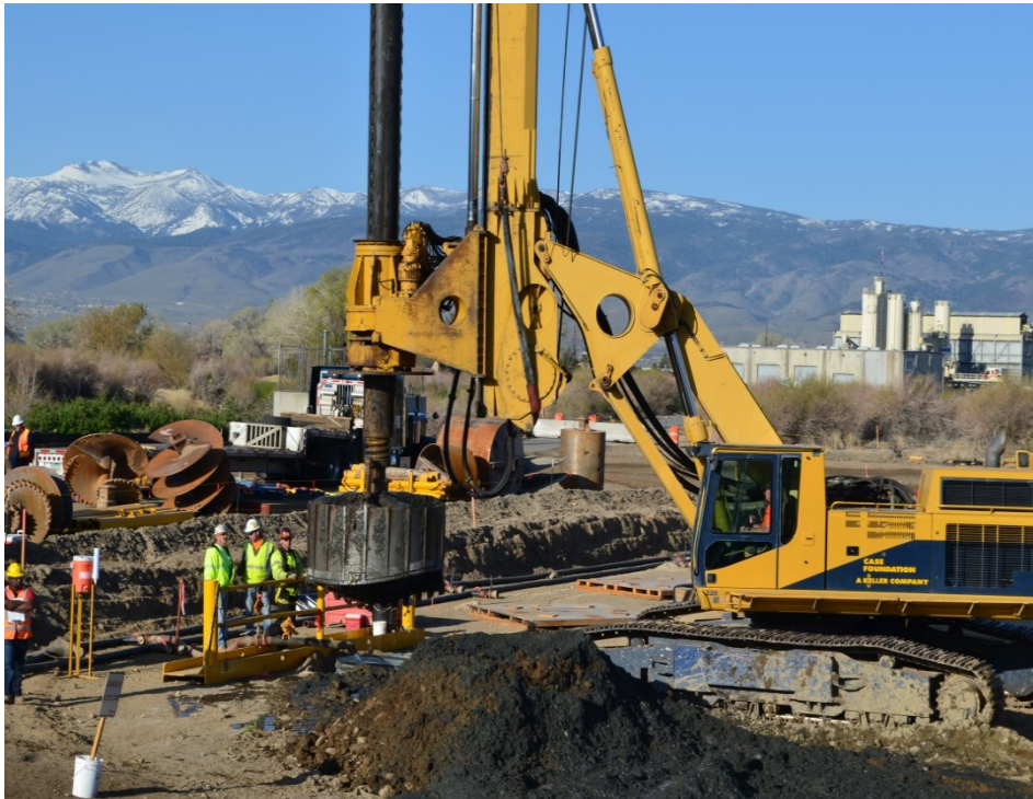
Piling, bridge over river
