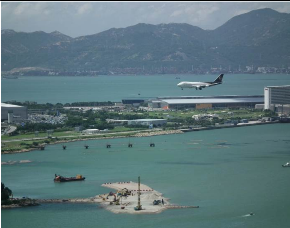
Ground improvement, airport link road
