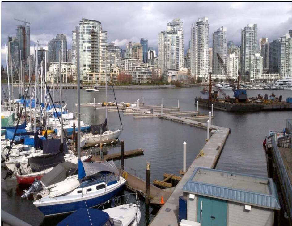
Piling, marina refurbishment
