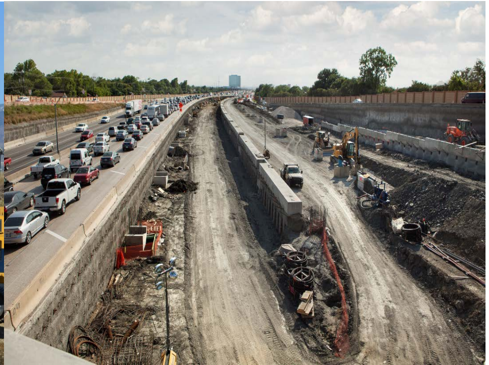
Earth retention, road toll lanes
