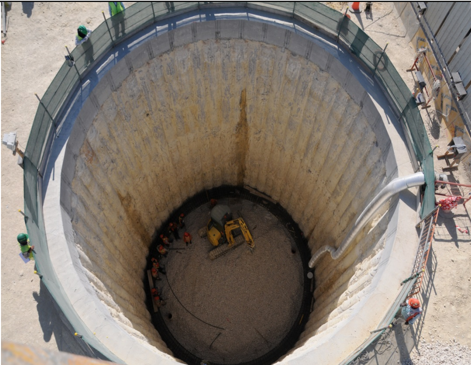
Piling, access shafts for sewage system
