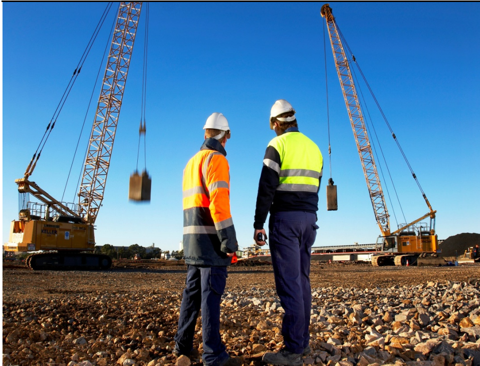
Dynamic replacement & soil mixing
