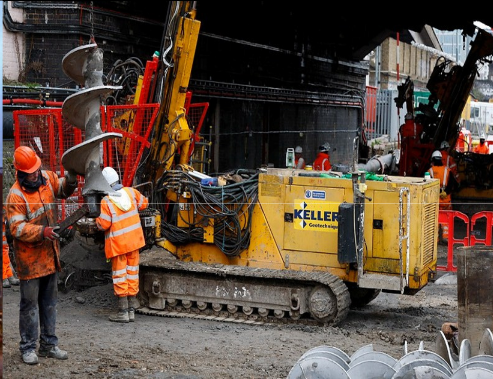
Minipiles Lord Hill's Bridge, London
