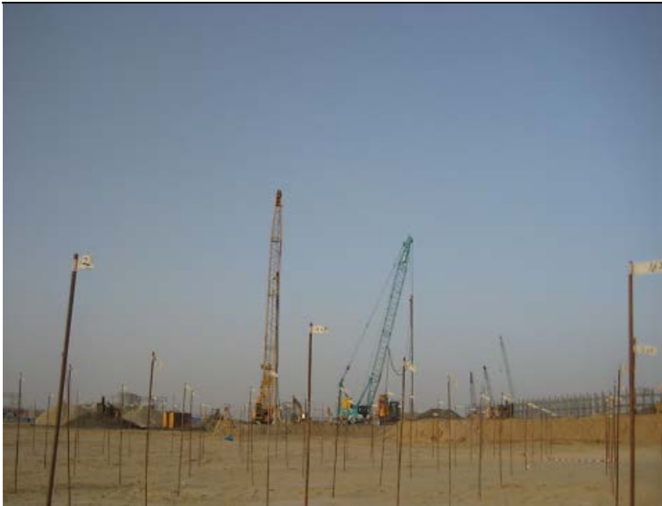
Vibro replacement, gas plant Al Jubail, Saudi Arabia
