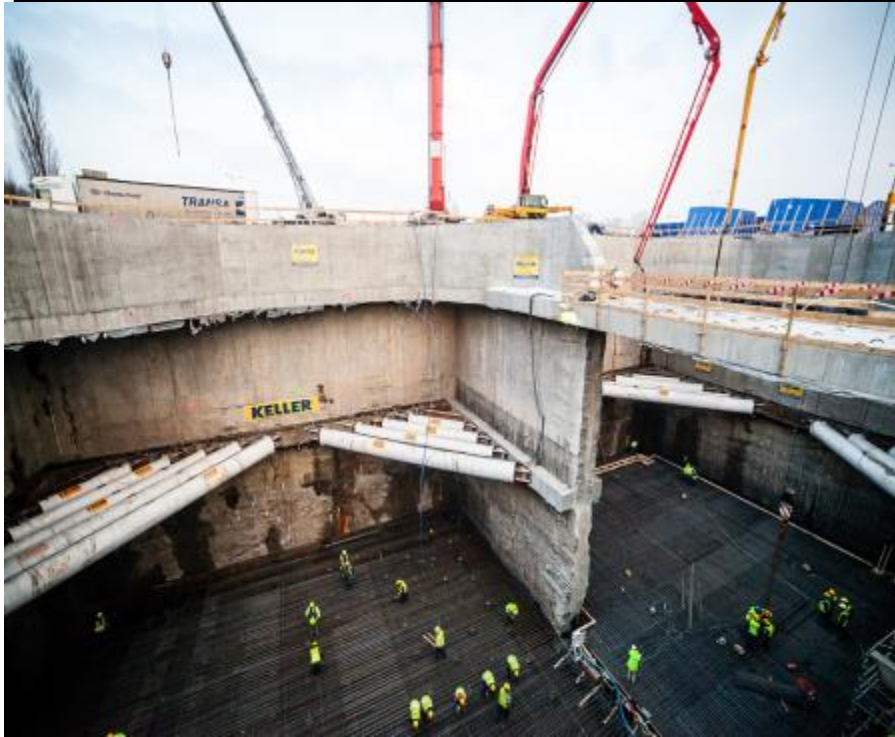
Excavated TBM chamber, road tunnel
