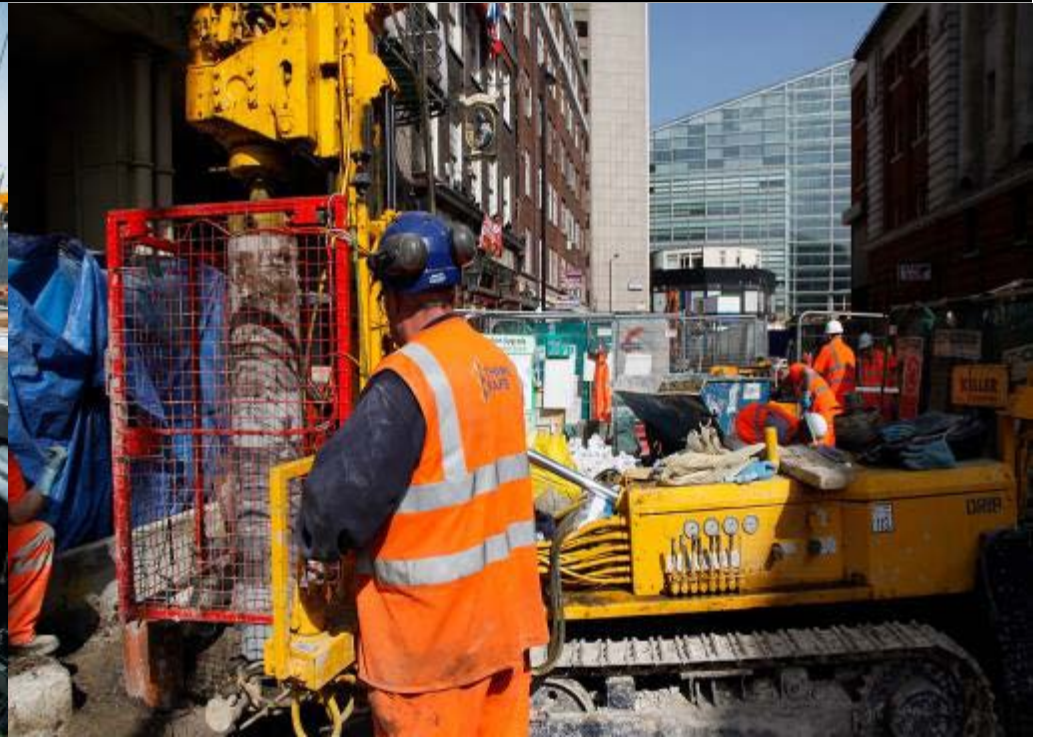
Specialty grouting, Victoria Station Upgrade
