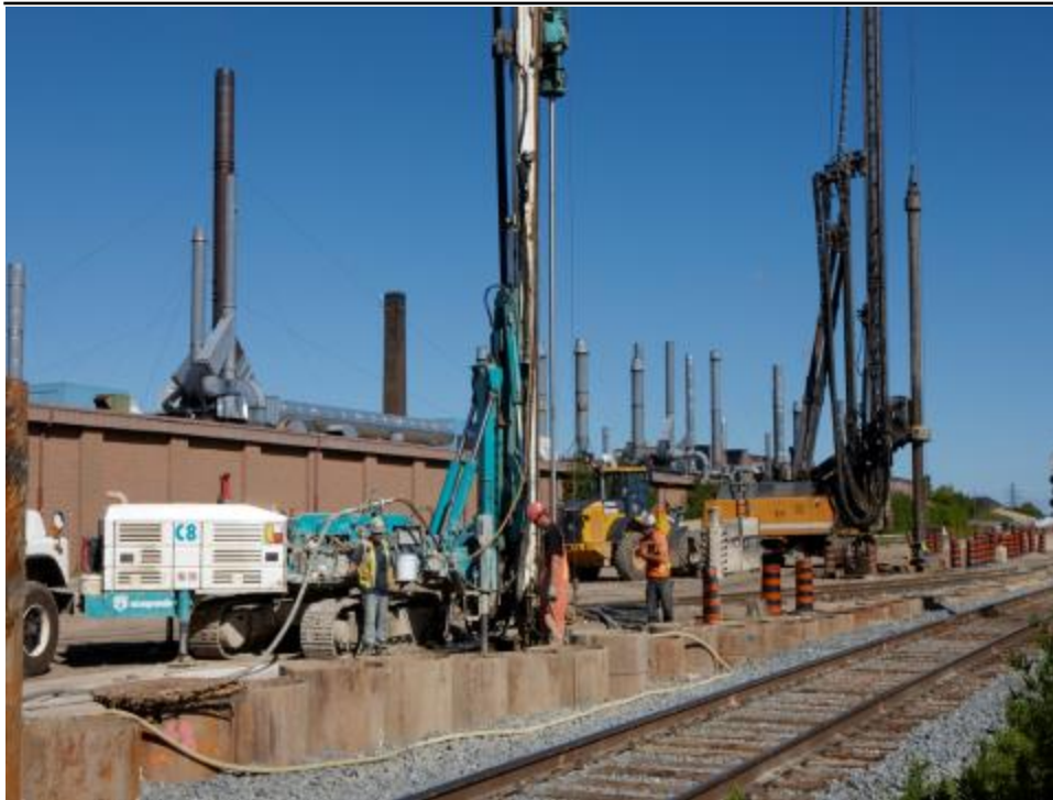
Jet grouting, rail grade separation project Toronto, Canada
