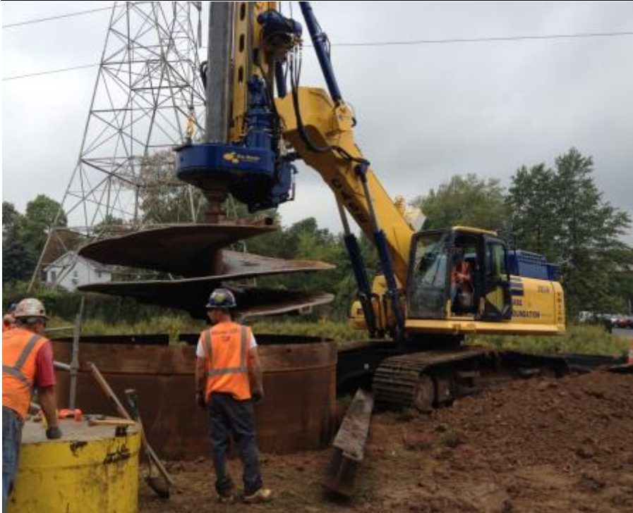
Piling, transmission line project New Jersey, USA
