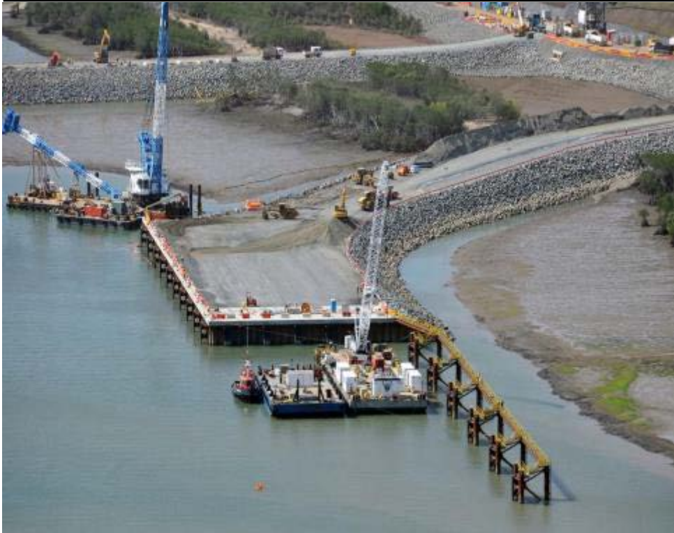
Off-shore piling, materials offloading facility Queensland, Australia
