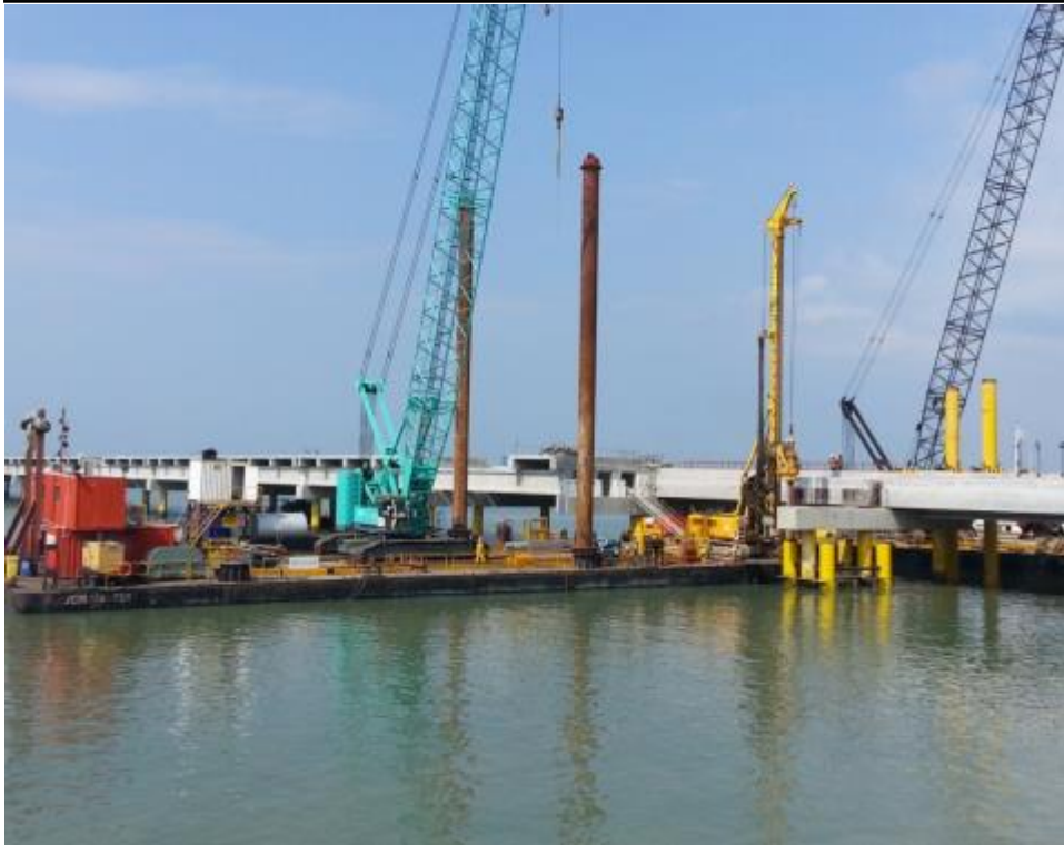
Off-shore piling, iron ore distribution facility
