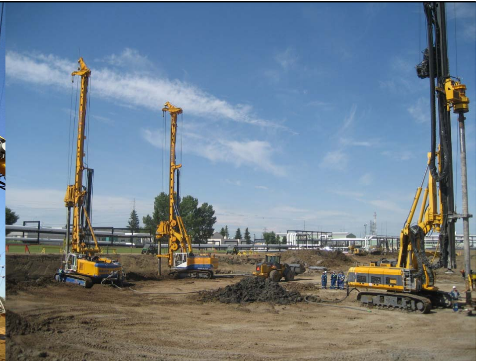
Soil mixing, tank expansion project
