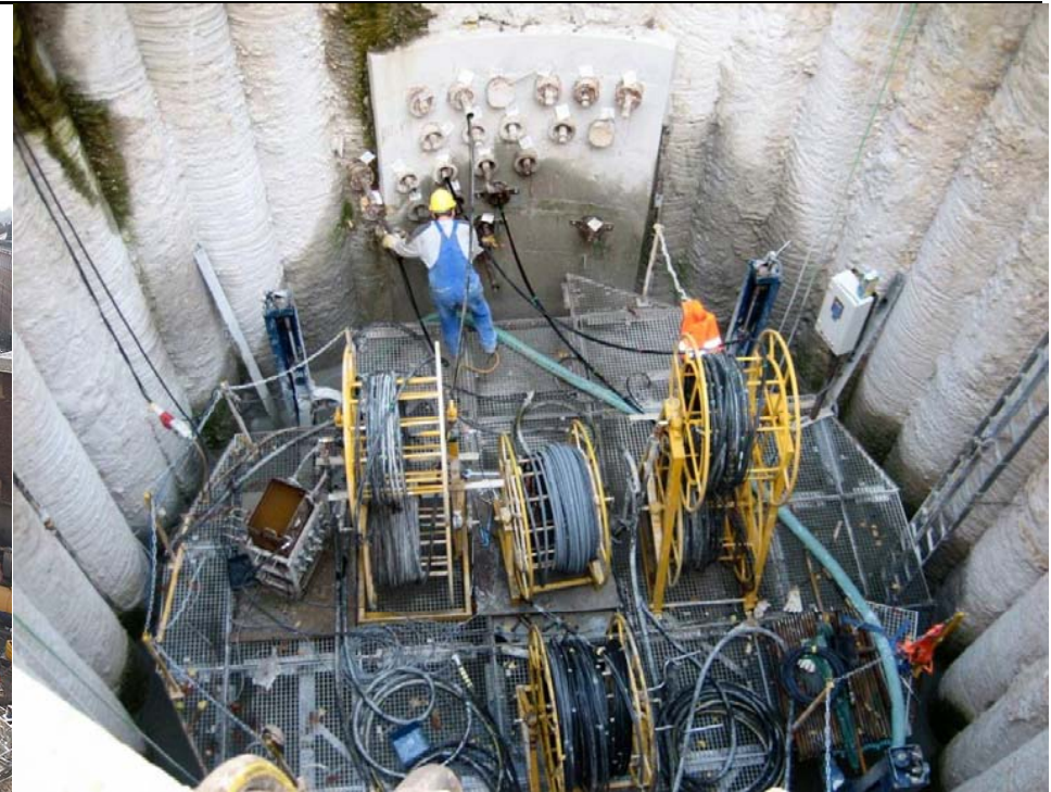
Compensation grouting, Crossrail
