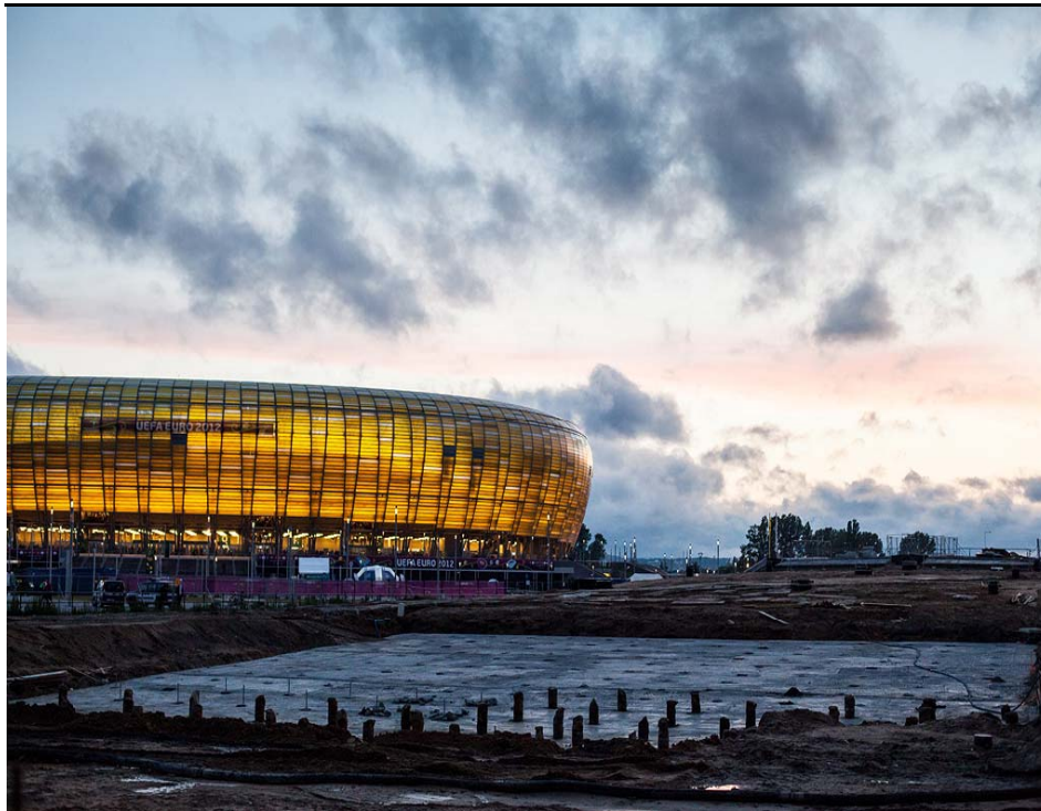
Soilcrete columns, road tunnel
