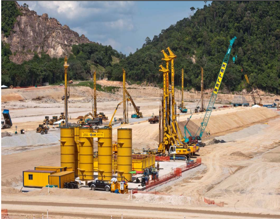
Piling and ground improvement, iron ore distribution facility
