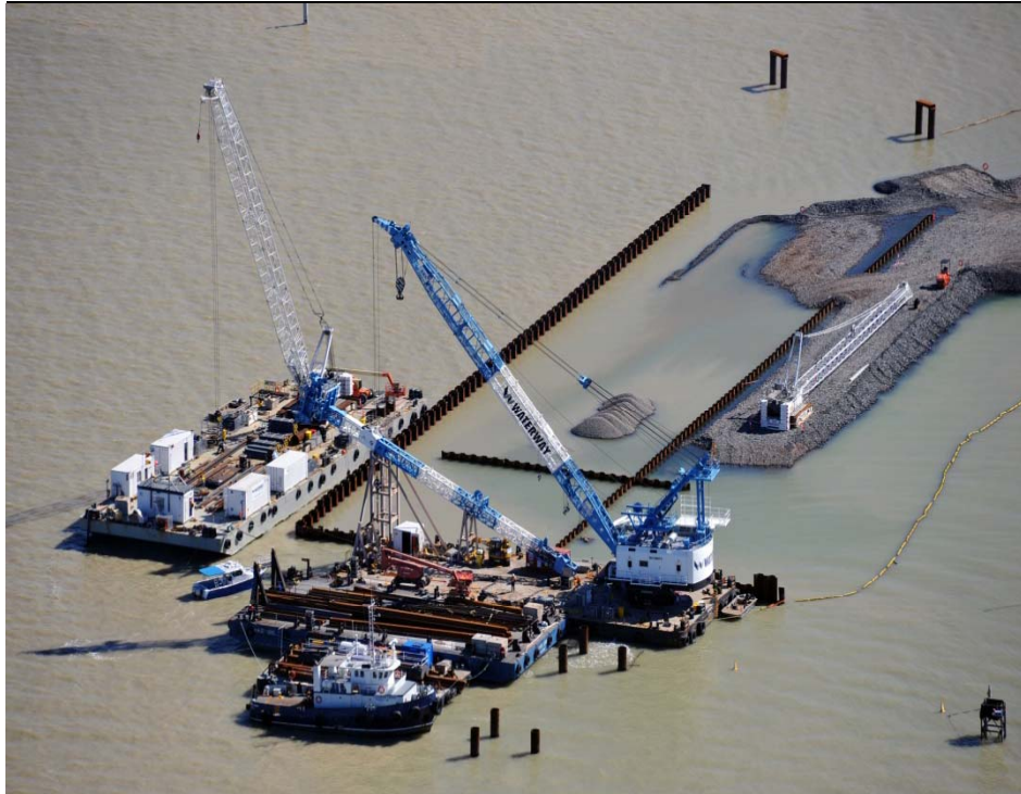
Offshore piling, materials offloading facility
