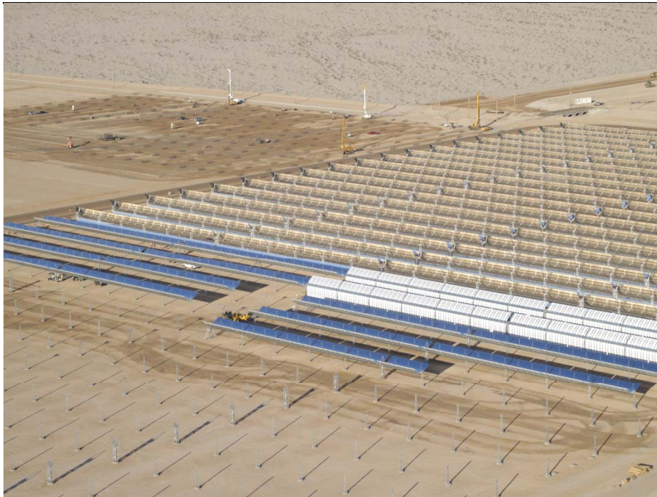
Piling, solar energy project
