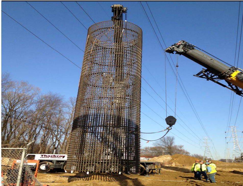
Piling, transmission line project
