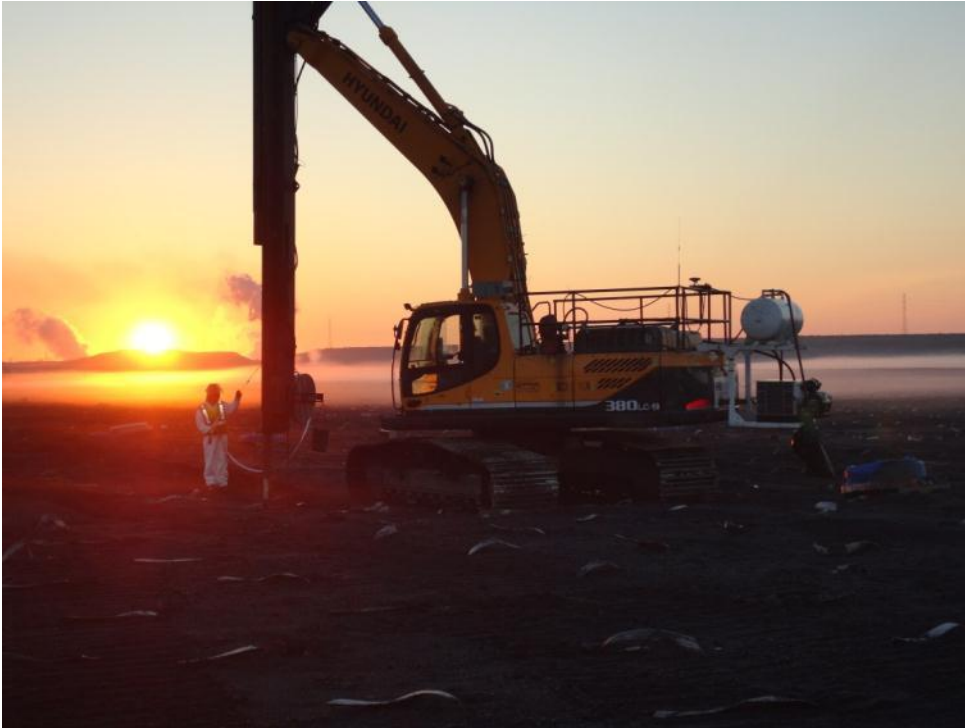
Hayward Baker on the $6m Suncor Wick Drain Contract
