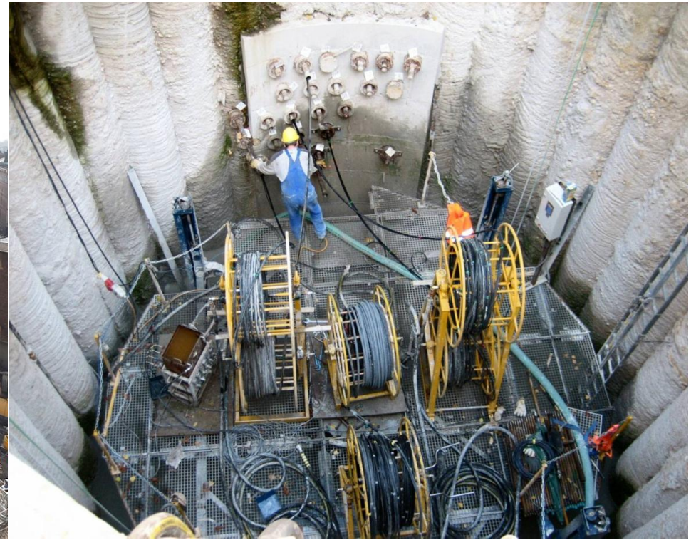
Compensation grouting, Crossrail London, UK Contract value: £20m (Keller's share)
