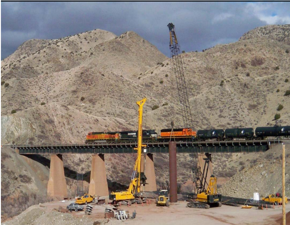
Double tracking of rail bridge Abo Canyon, New Mexico
