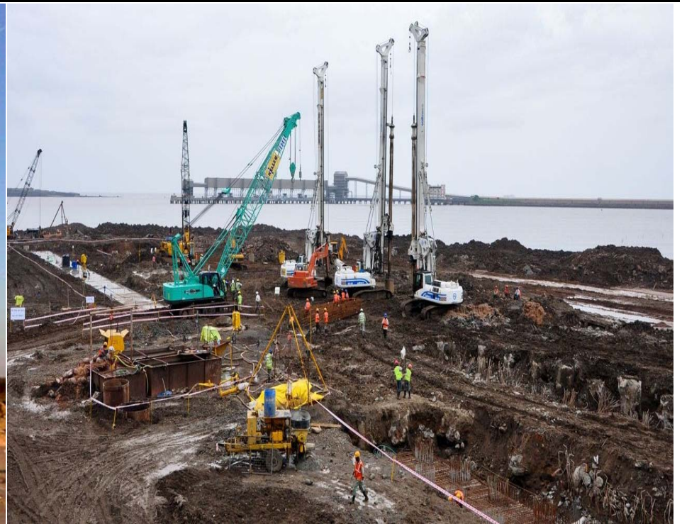
Foundations for fabrication yard
