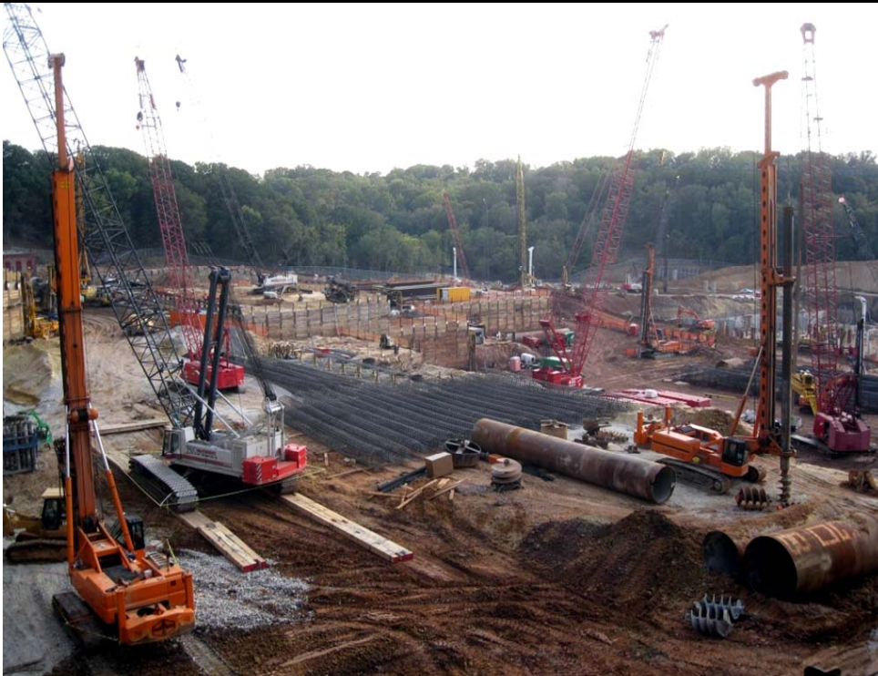
Slope protection for Government building Washington DC
