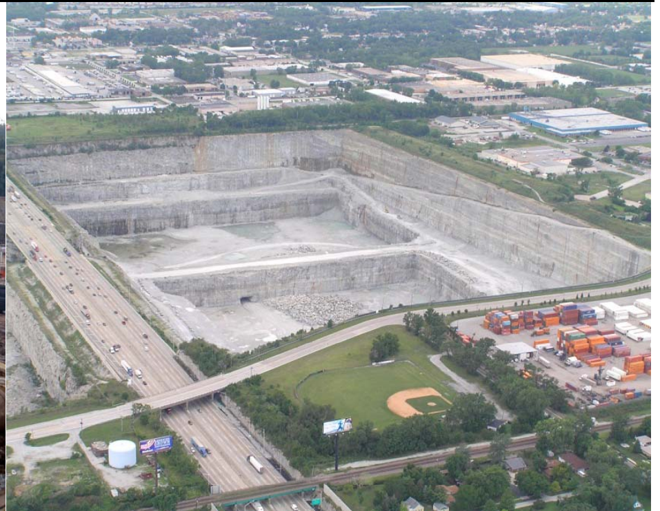
Grouting at Thornton Composite Reservoir Chicago, Illinois
