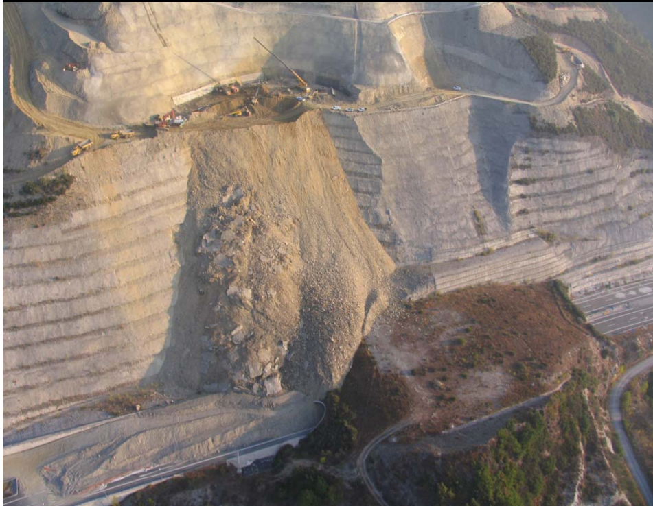
Emergency landslide repair
