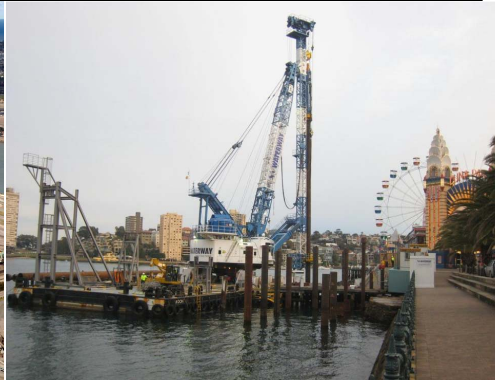
Wharf upgrade Sydney, NSW
