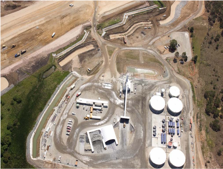
Infrastructure for grouting of disused mine workings, Queensland Engineering support from three continents
