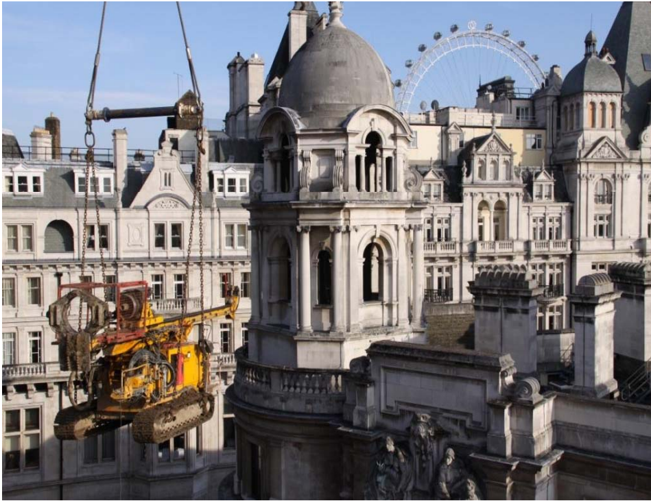
Refurbishment of Corinthia Hotel, London
