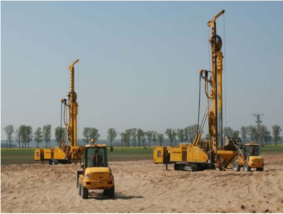
Eastern Europe New A1 motorway south of Gdansk, Poland Ground improvement
