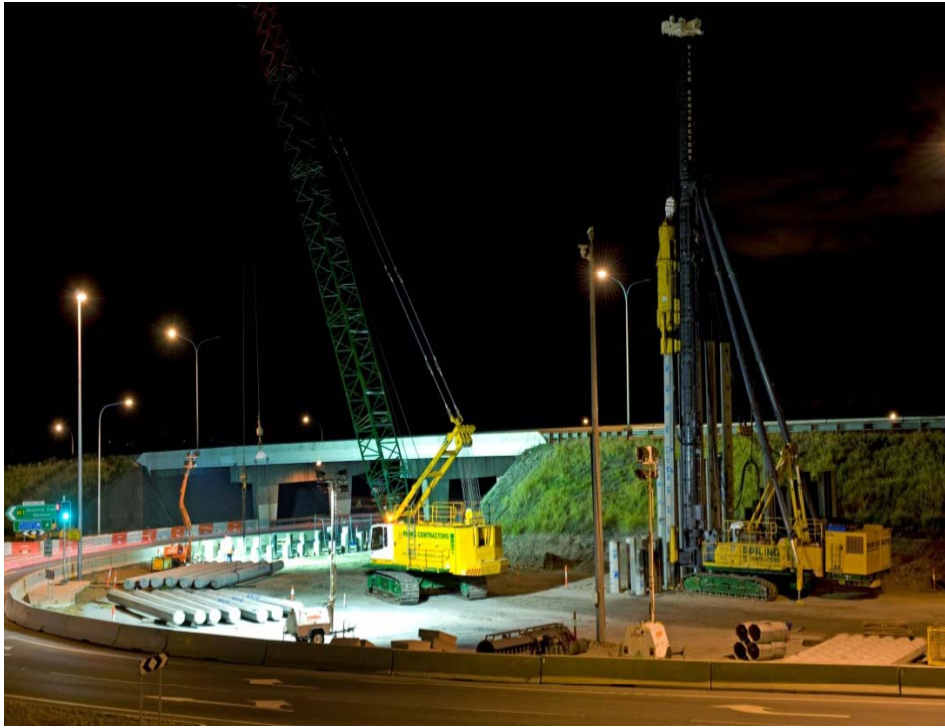
Piling work on road infrastructure, Brisbane
