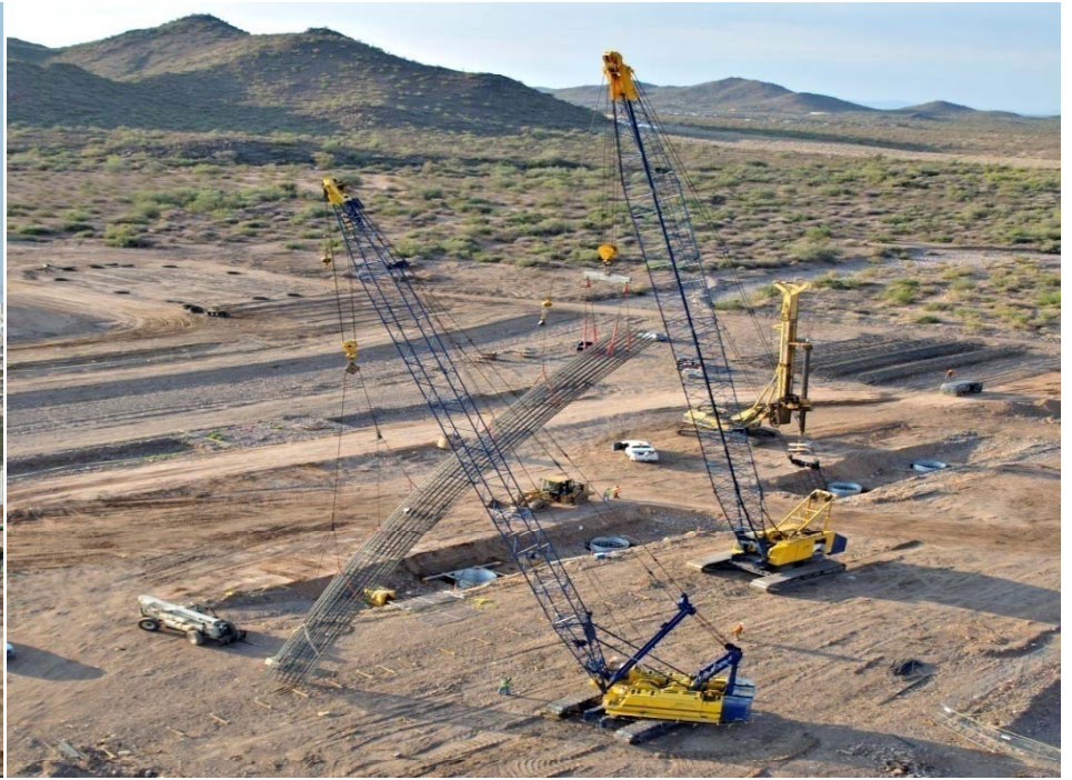
Route 303 Outer Loop Freeway, Arizona Bored piling for nine new bridges
