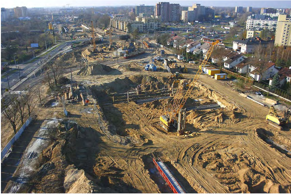
Eastern Europe New S8 Expressway, Warsaw Diaphragm walls and Jet grouting
