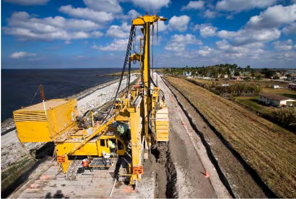
Lake Okeechobee, Florida Strengthening of dyke using TRD technology
