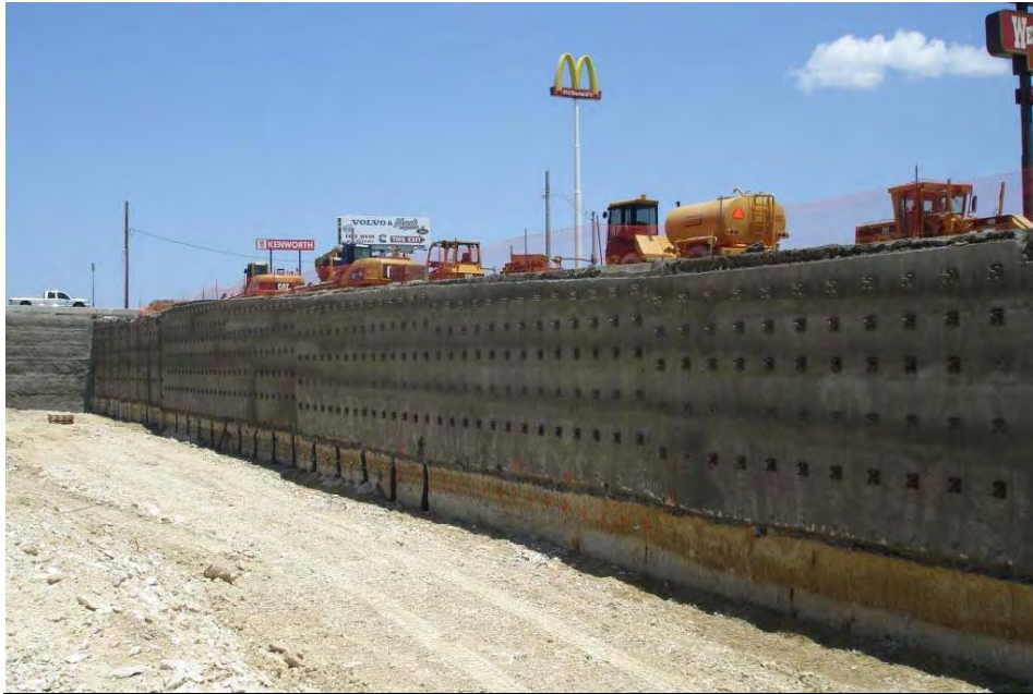
Dallas Area Rapid Transport System, Texas Retaining wall with soil nails
