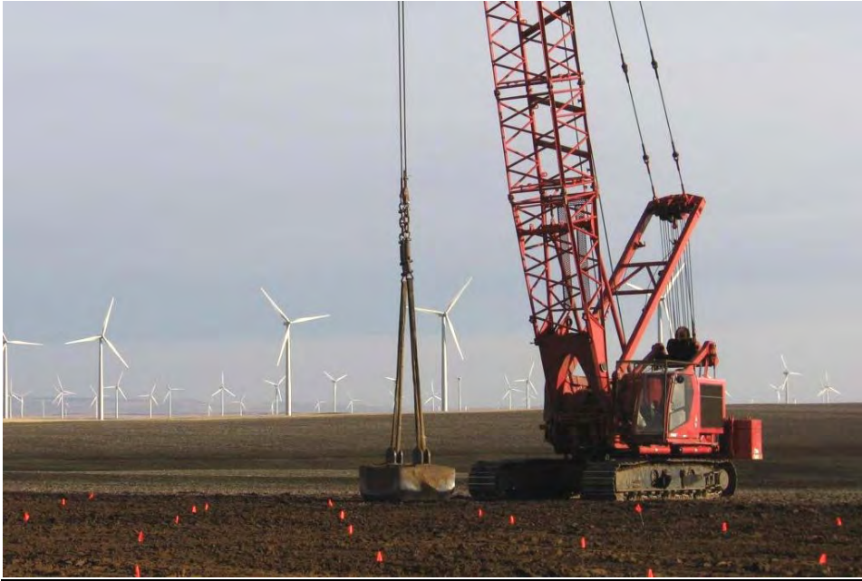
Wind farm, Oregon Dynamic compaction
