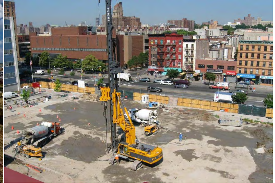
Extension at hospital, New York Compaction grouting to densify soils
