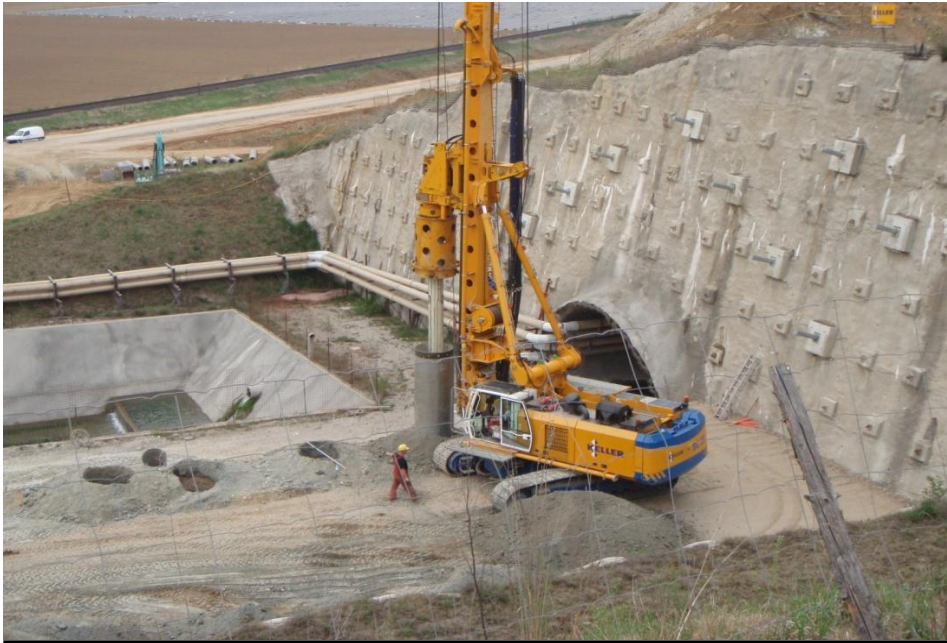
New railway tunnel, Southern Austria Bored piles, anchors, nails & shotcrete
