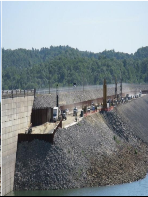
Remedial work at the Wolf Creek Dam, Kentucky Drilling and grouting to cut off water seepage
