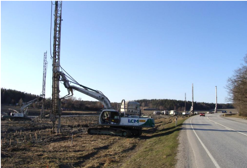
Road upgrade near Stockholm, Sweden Ground improvement using dry soil mixing
