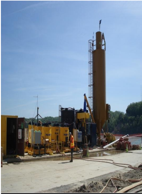
Remedial work at the Wolf Creek Dam, Kentucky Drilling and grouting to cut off water seepage
