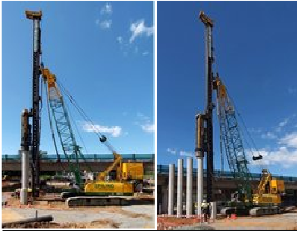
Caboolture bypass, Brisbane, Queensland Piling Contractors installing driven piles
