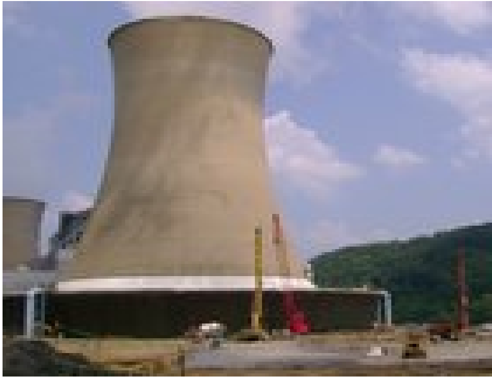
Piling at power plant, West Virginia McKinney & Case working together
