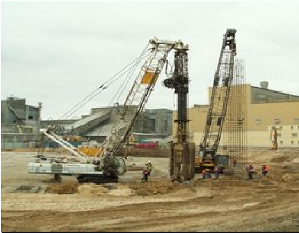
Cement plant, South East Poland Foundations for a new clinker silo
