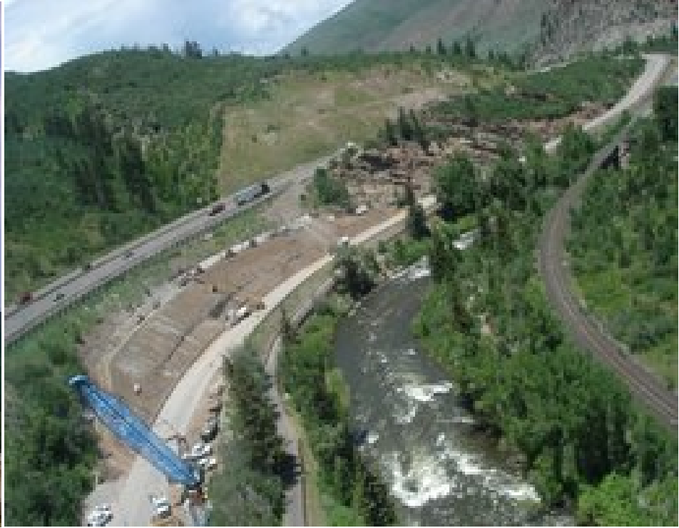
Emergency repair on road embankment, Colorado Anchors, soil nails and minipiles
