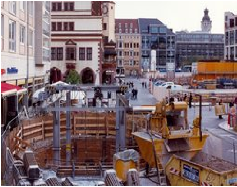
City tunnel project, Leipzig, Germany Compensation grouting to protect buildings
