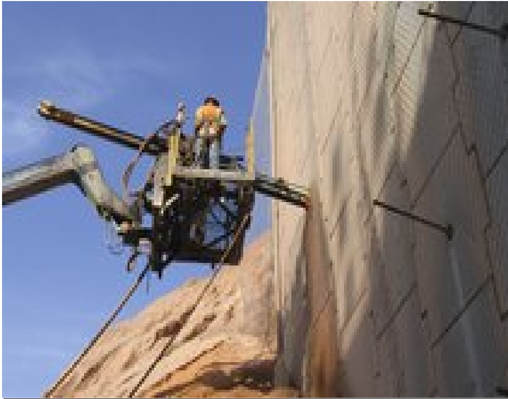
Copper mine, Arizona Emergency wall repair using anchors
