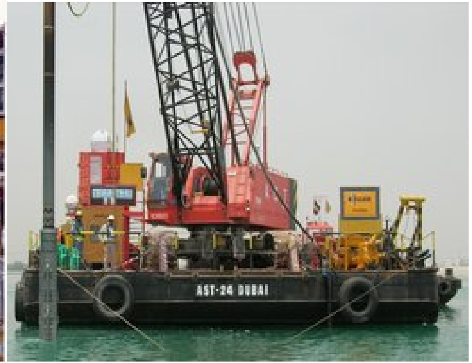
Al Raha Beach Resort, Abu Dhabi, UAE Onshore & offshore ground improvement
