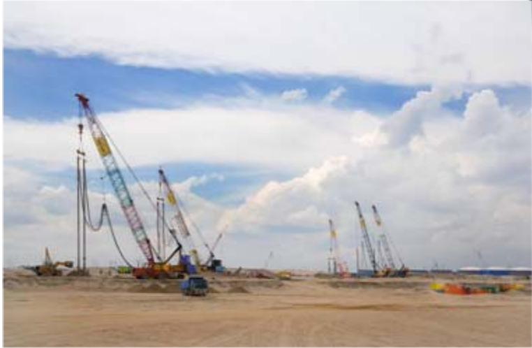
Vibro compaction in progress at Universal Terminal, Jurong Island, Singapore
