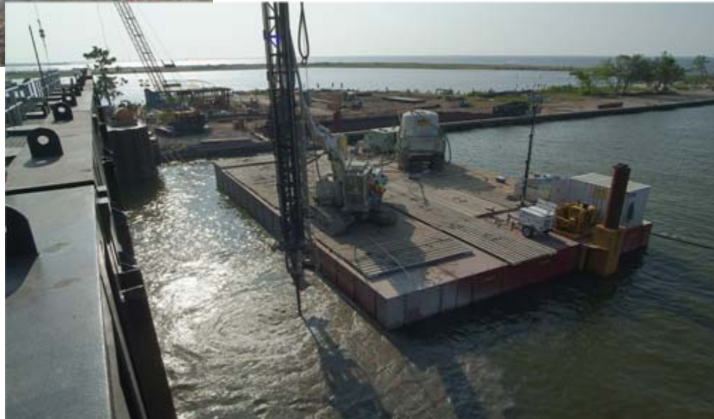
Hayward Baker Dry soil mixing & jet grouting New flood defence gates New Orleans, Louisiana
