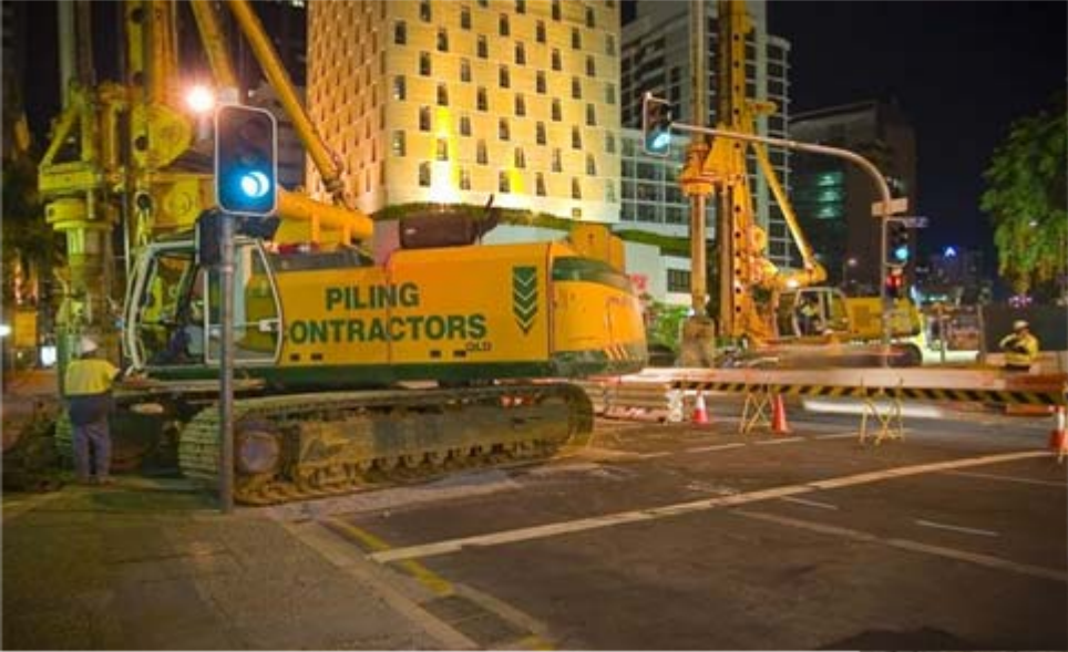
Bored piles Inner northern busway Brisbane
