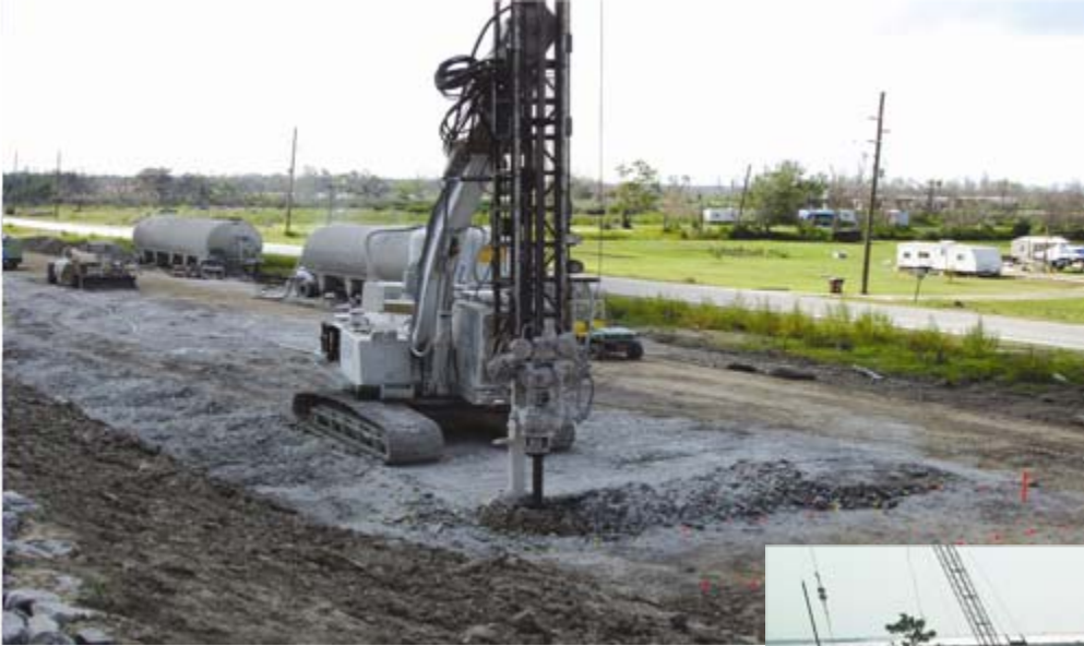
Hayward Baker Dry soil mixing Levee reconstruction Buras, Louisiana
