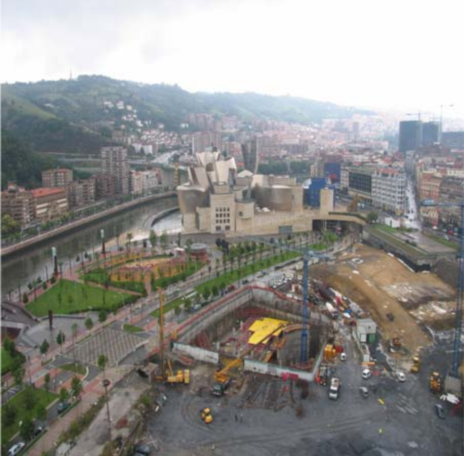
Keller-Terra, ground improvement with stone columns, Campa de los Ingleses, Bilbao
