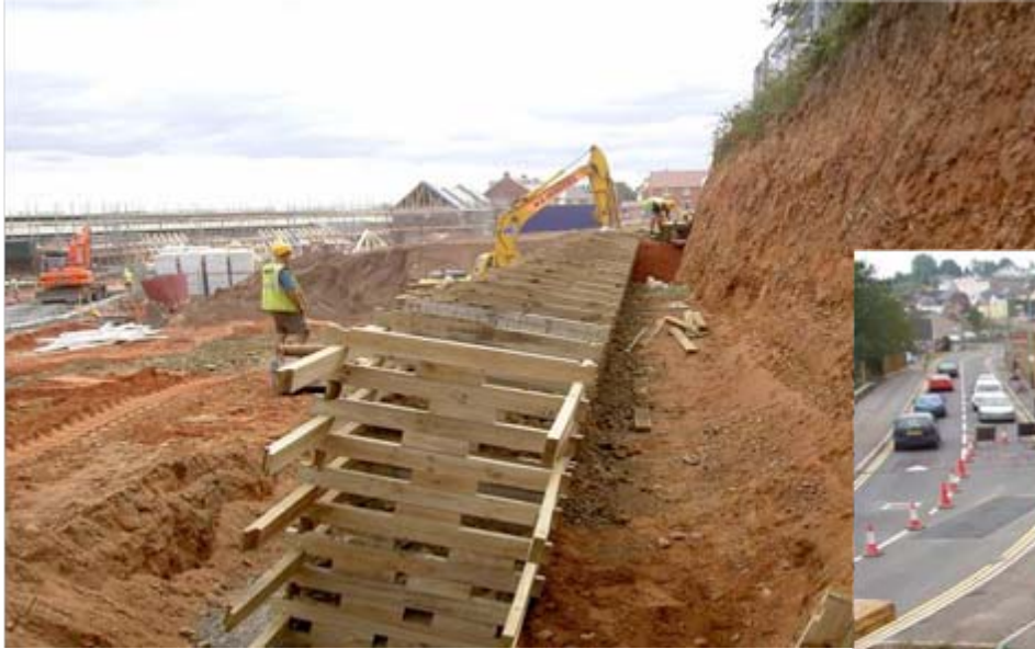
Timber crib wall during construction
